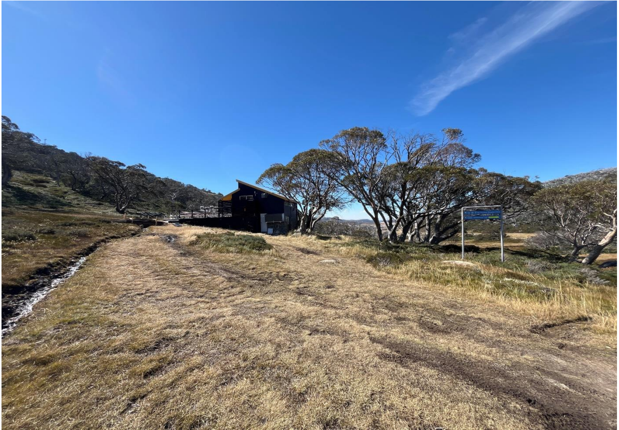
Photo 5: The existing vehicle access will be formalised by the addition of 150 mm of gravel over the existing surface which comprises bare ground and exotic grassland.
